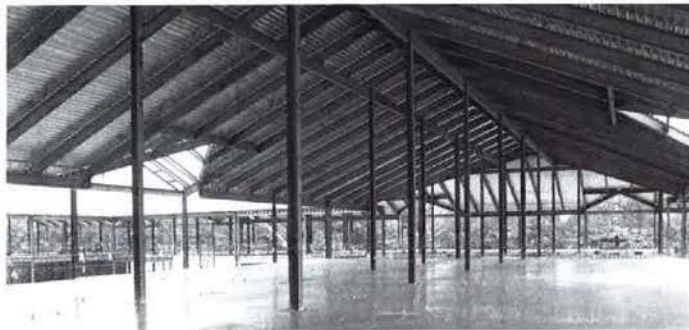
Second-floor classrooms on north wing
